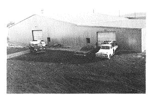
A new warehouse has been erected south of the Shot Plant. The all-steel structure contains 12,000 square feet of storage area and is now being used for stocking abrasives and extra production parts.
